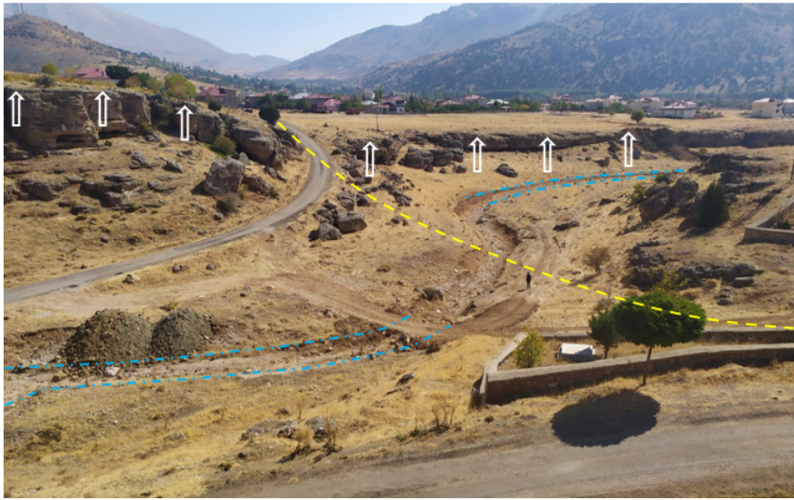
Figure 8. Topographic elevation difference and stream offset in Barış village (looking towards SE). The yellow dashed line shows the fault line, the blue dashed lines show the offset of channel edges, and the white arrows show the elevation difference.
