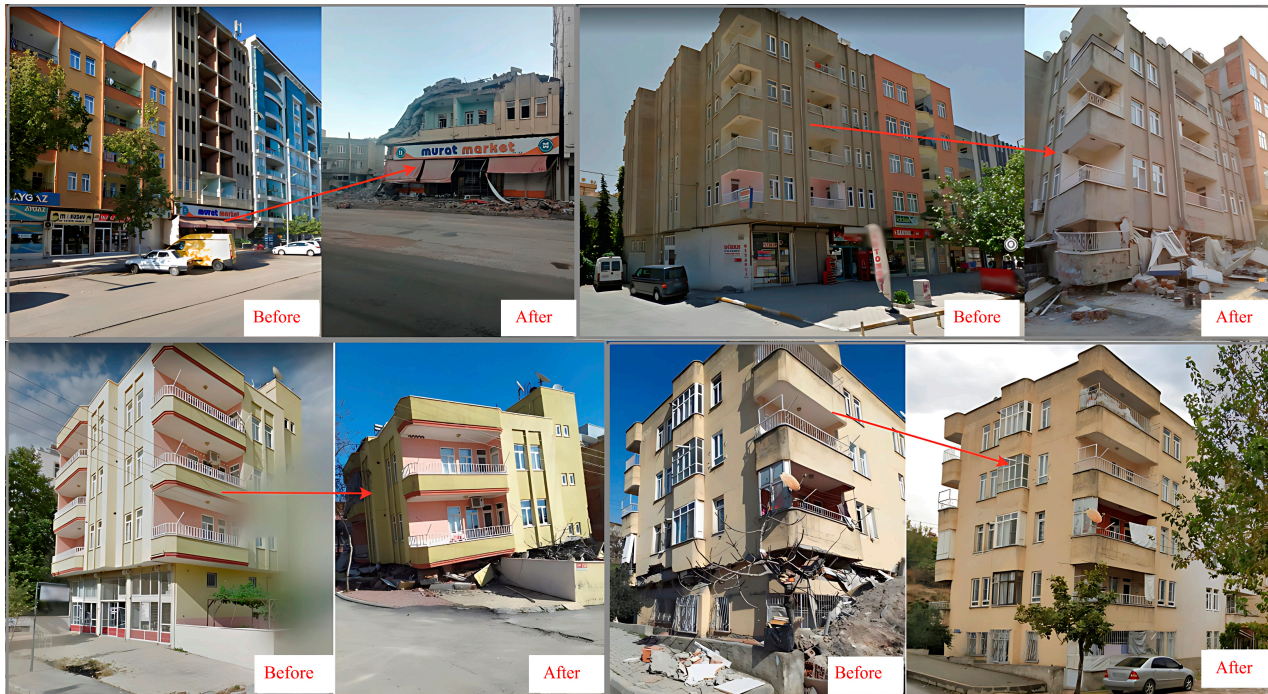
Figure 6. Comparison of some RC building examples before and after the earthquake.
