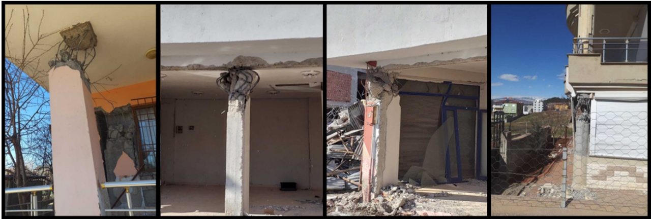
Figure 5. Plastic hinges occur in the upper-end regions of the column.
