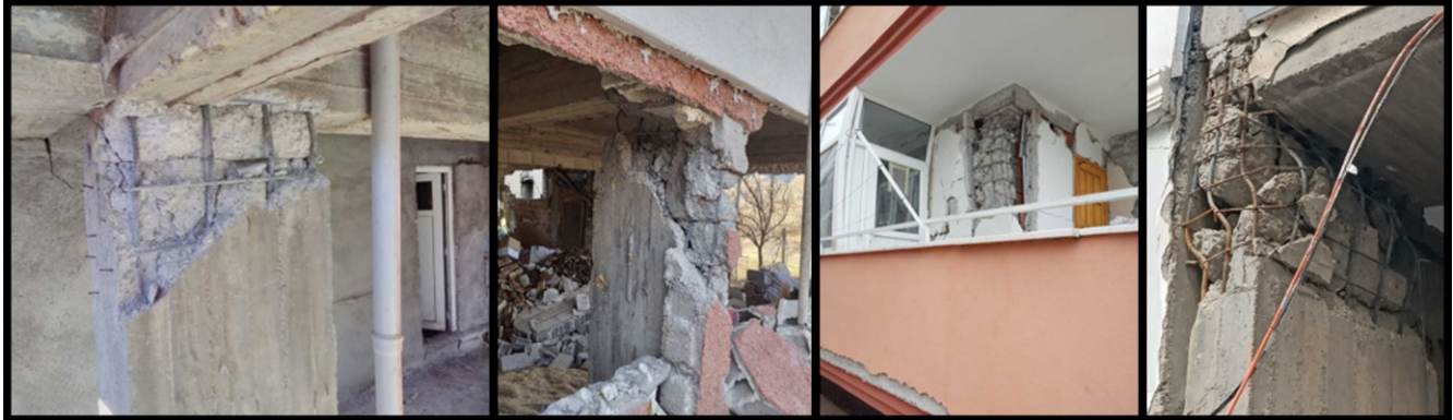
Figure 13. Use of different types of reinforcement.
