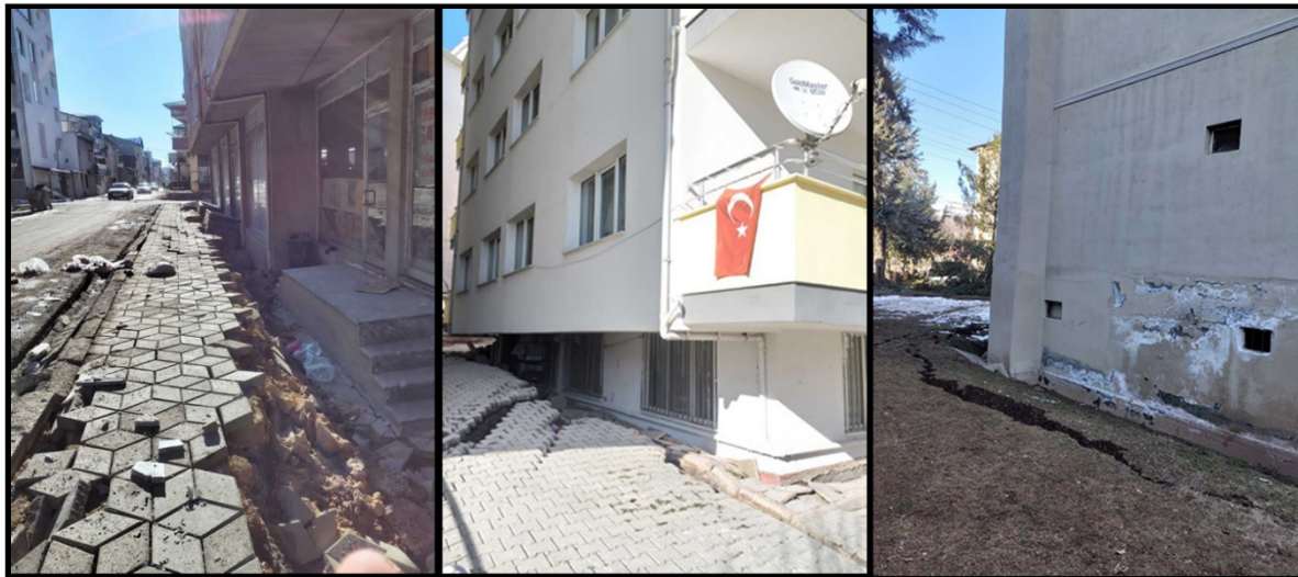
Figure 7. Damage caused by liquefaction.
