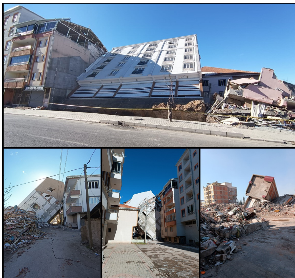
Figure 8. Examples of the lack of sufficient foundation depth.
