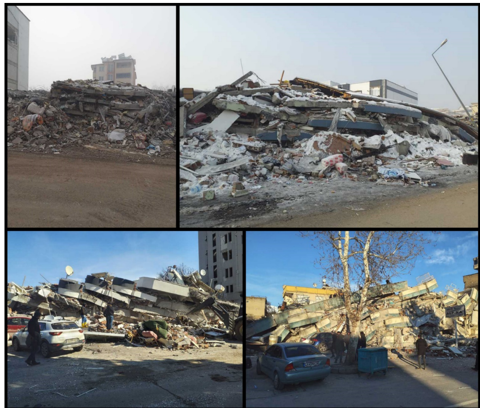
Figure 11. Examples of pancake-type collapse.
