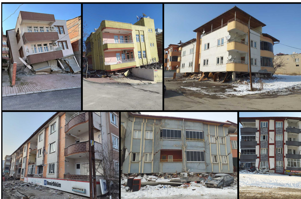
Figure 10. Examples of buildings with partially or completely collapsed ground story due to soft stories.
