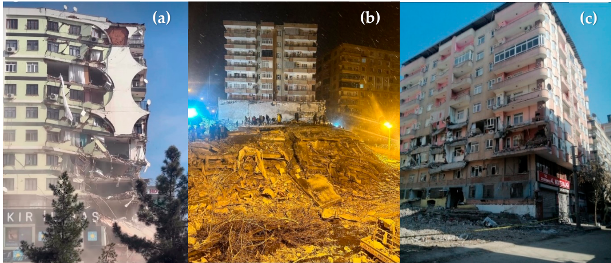
Figure 4. Structures that collapsed during the mainshock on 6 February 2023: (a) Galeria Business Center (Yenişehir district), (b) Serin-2 Apartment (Bağlar district), and (c) Yoldaş Apartment (Bağlar district).
